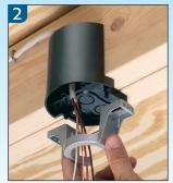
2. Position mounting bracket over locator posts to assure proper position. Pull wires through KO.
